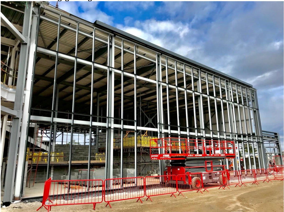
Leisure Building glazing frame installation:
