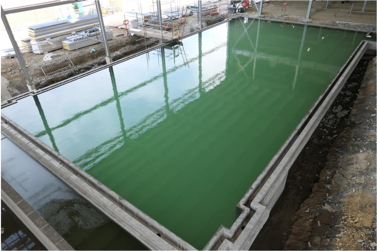
Main swimming pool in the Leisure Building – 1 st water testing process:
