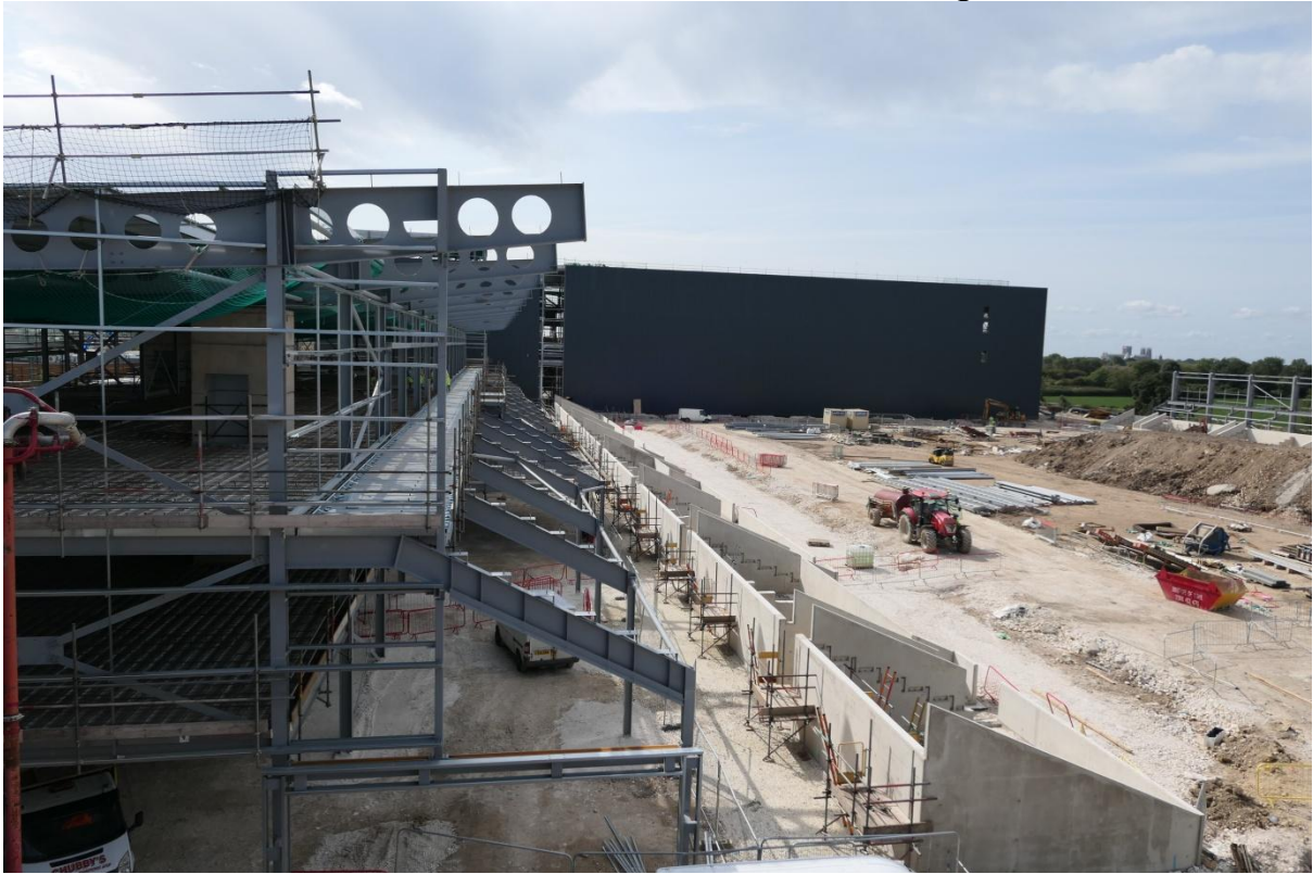
Stadium Main / East Stand, view from Leisure Building Roof:
